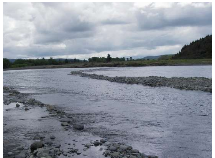
River diversion and the weir across the river in the background.
